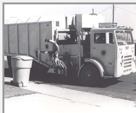
The Automated Sideloader Scottsdale 1974
